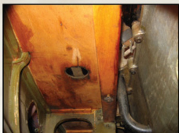
Underneath the right engine bearer. Note the interior grey green protective paint on the lower surfaces of the engine bay.
