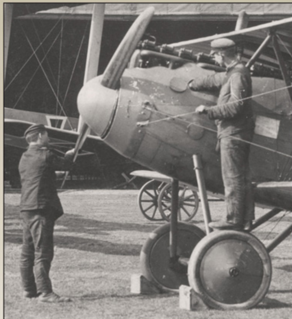
∨ A nice diorama idea as ground crewmen prepare Albatros D.V D.4640/17 for flight at Mariakerke. Note the 180ps Daimler-Mercedes D.IIIa engine, additional drag cables and rigging guide fixed to the side of the fuselage.
