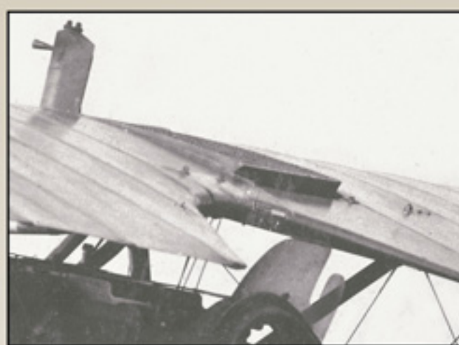
Note the aileron pulley cover and painted Daimler-Mercedes radiator of this unidentified Albatros D.V.
