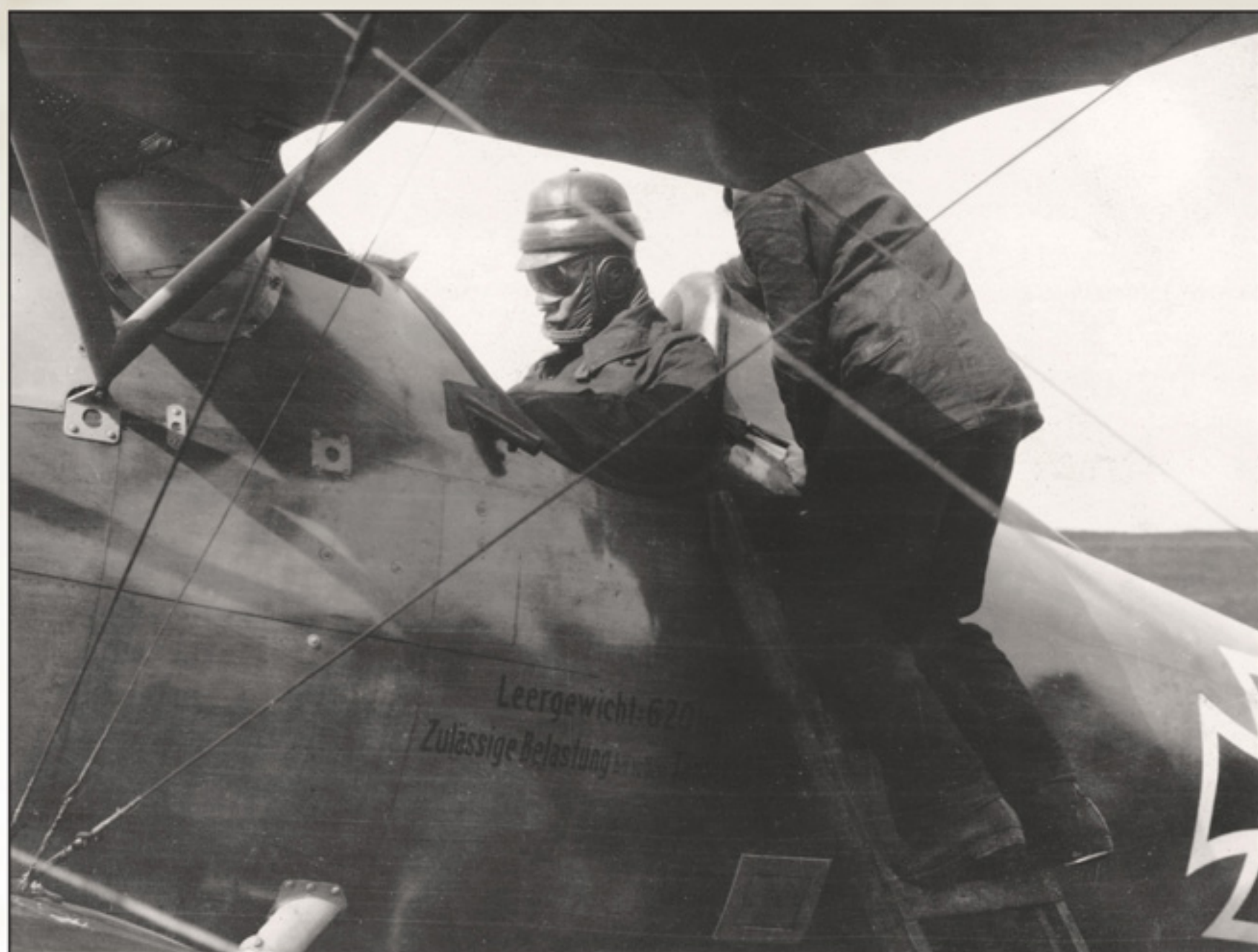
An unidentified pilot wrapped up for protection from the elements prepares for a flight in this early Albatros D.V. Note the headrest, placement of the flare pistol and the dark appearance of the varnished wooden fuselage. All metal fittings remain
