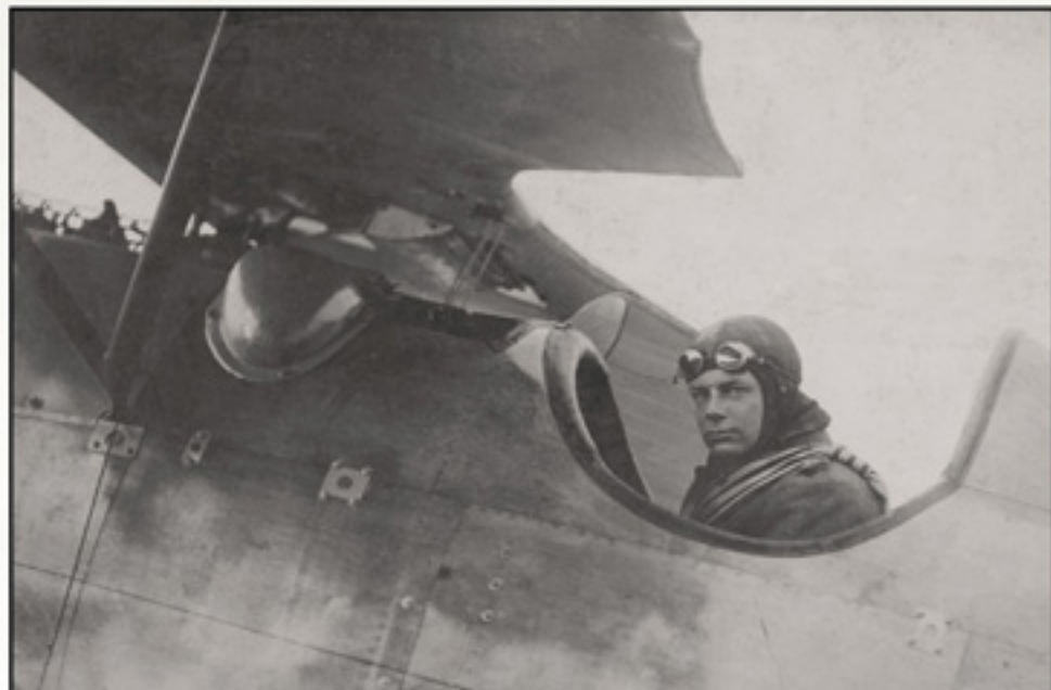
An unidentified pilot sitting in an early Albatros D.V. Note the head rest, LMG 08/15 empty belt chute fairing, aileron cables entering the upper wing and the unusual 'scoop' fixed under the radiator to aid cooling and multi coloured 4 point safety harness, possibly red and white.
