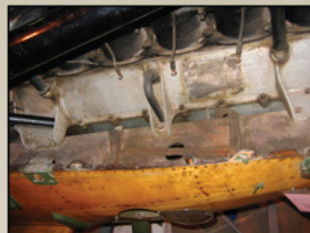
Right engine bearer showing the mounts for the oil tank.
